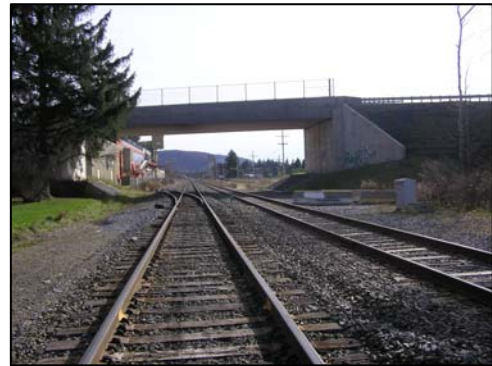
Rail line passing under Route 6 in Port Allegany
