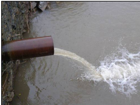
Stormwater discharge following a significant rainstorm near Foster Township Park
