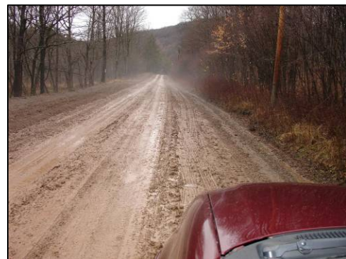
Improperly designed dirt and gravel roadways can increase the amount of sediment washed into nearby waterways (Source: Potter County Conservation District)
