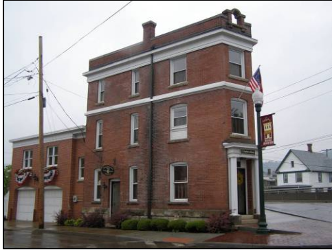
Rufus Barrett Stone house is uniquely positioned between Tunungwant Creek, Boylston Street, and East Washington Street
