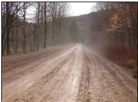
Improperly built and managed dirt and gravel roadways increase the amount of sediment entering streams via runoff following a precipitation event (Source: Upper Allegheny Watershed Association)
