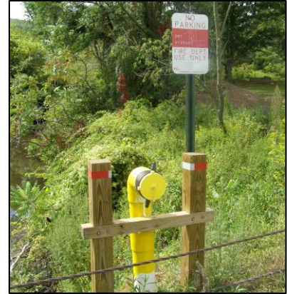
Dry hydrant located along an area waterway
